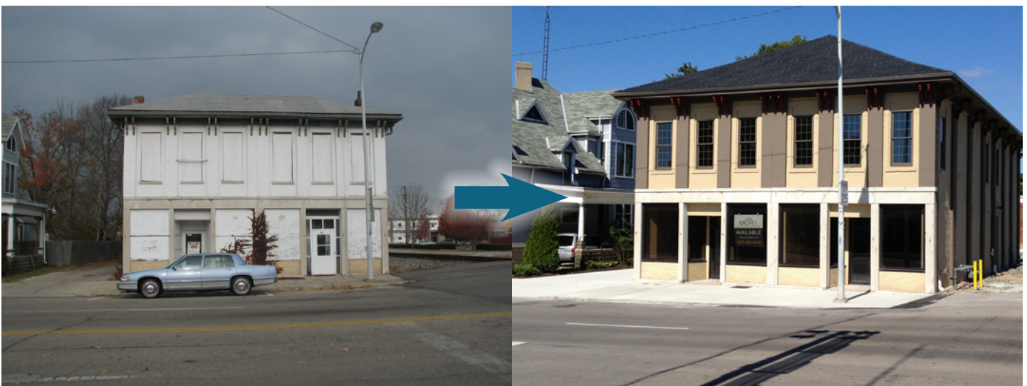
Troy Community Works rehabilitated the East Gate building into productive use.
