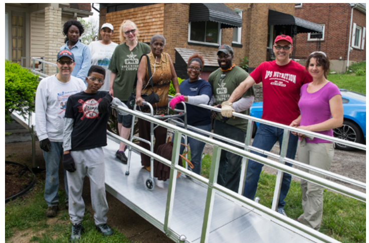
People Working Collaboratively performs repairs to provide safe access to homes.
